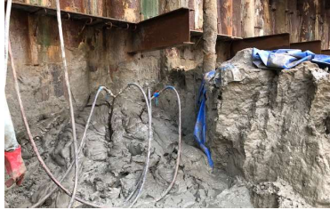
Needle grouting
