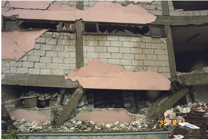
(Pancaking collapse of soft storey 1999 Izmit earthquake)
