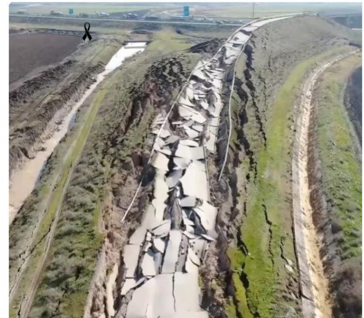
An extraordinary lateral spread in an embankment, triggered by the 2023 Turkey-Syria earthquakes. Image from a video posted to Twitter by @Sabah.
