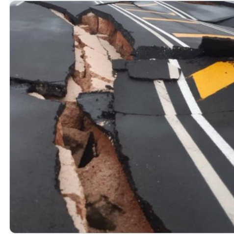
Earthquake Cracks Occured at Sultansuyu Dam in Malatya
