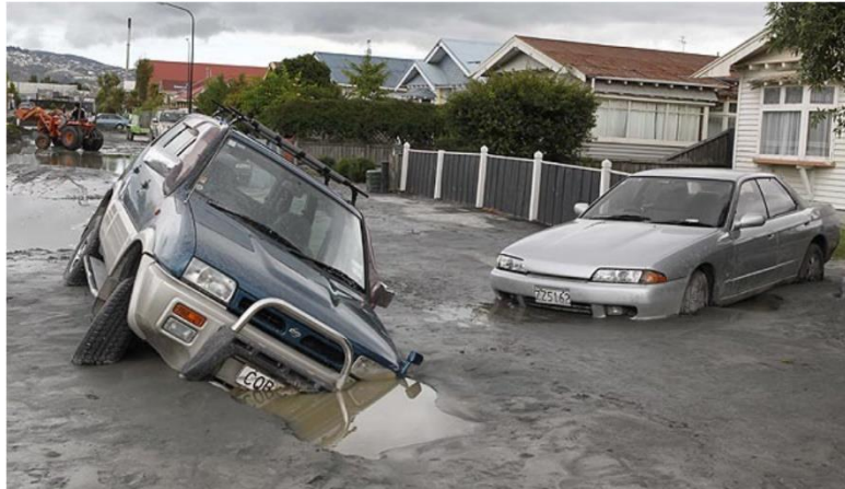
Soil liquefaction after the New Zealand Christchurch Earthquake in 2011. (Source: Stuff.co.nz)
