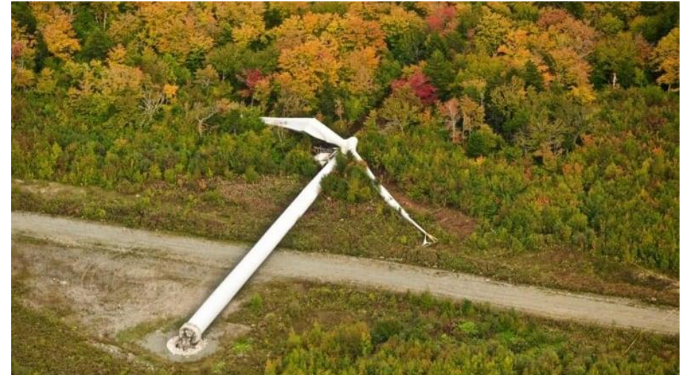
Foundation collapse
